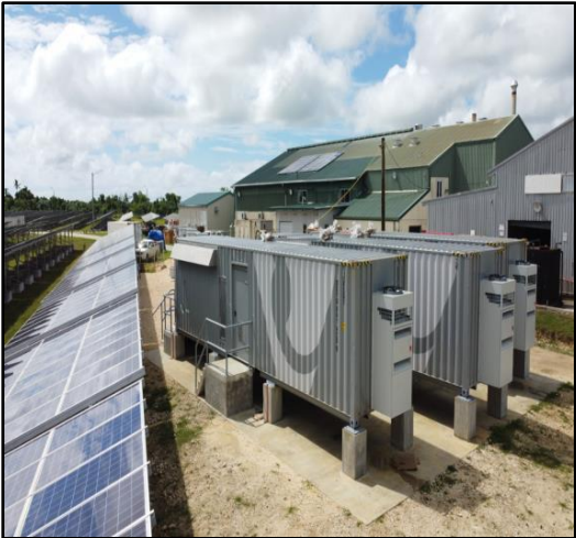
Figure 17. Battery energy storage system at the Popua power station.
