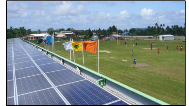
Figure 23. The first grid-connected solar PV system in Tuvalu (40 kW).
