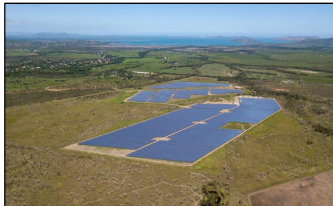
Figure 12. The Helio Boulouparis 2 Solar Park (16 MW, 10 MWh ESS).
