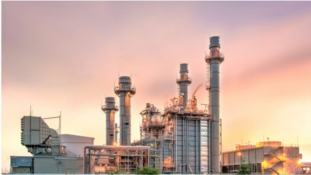
FIGURE 15. H 2 GAS BASED POWERPLANTS. H 2 FUEL-READY GAS TURBINES ARE BEING INSTALLED IN RETROFITTED OR NEWLY BUILT NATUREL GAS-BASED POWERPLANTS. FOR EXAMPLE, THE ABOVE FIGURE SHOWS THE TALLAWARRA NATURAL GAS POWERPLANT IN AUSTRALIA, WHERE A HYDROGEN-READY TURBINE HAS BEEN INSTALLED THAT WILL OPERATE WITH A 5% H 2 FUEL BLEND BY 2025 AS A DEMONSTRATION PILOT PROJECT.
