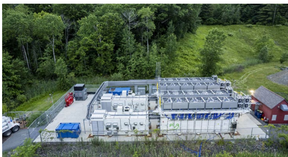
FIGURE 11. STATIONARY FUEL CELL SOLUTIONS FOR POWER GENERATION. IMAGE COURTESY OF PLUG POWER.
