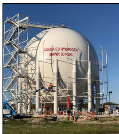
FIGURE 8. LIQUID H 2 IS STORED IN SPHERICAL CRYOGENIC TANKS. IMAGE COURTESY OF NASA.
