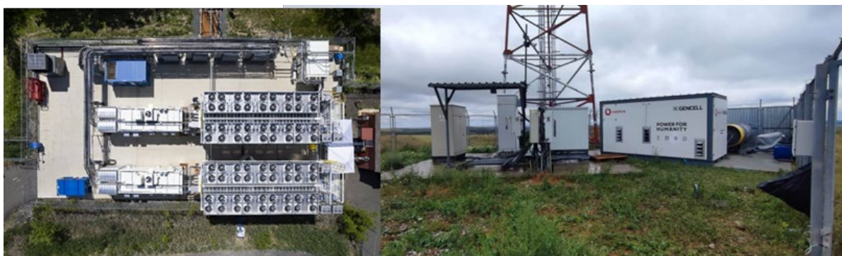
FIGURE 13. EXAMPLES OF HYDROGEN FUEL CELL APPLICATIONS AS A BACK-UP POWER SOURCE FOR CRITICAL INFRASTRUCTURE. FUEL CELLS ARE BEING INCREASINGLY USED FOR THEIR RELIABILITY WHICH IS IMPORTANT FOR APPLICATIONS LIKE DATA CENTRES (FUEL CELL INSTALLED AT A MICROSOFT DATA CENTRE IS SHOWN ON THE IMAGE ON THE LEFT) AND FOR TELECOMMUNICATION TOWERS (AS SHOWN ON THE IMAGE ON THE RIGHT).
